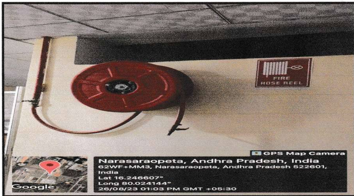
Fig: Wheel grid in the corridor
